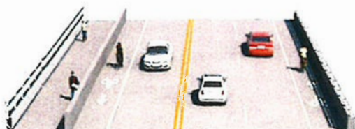
Causeway Drive - Banks Channel Bridge
