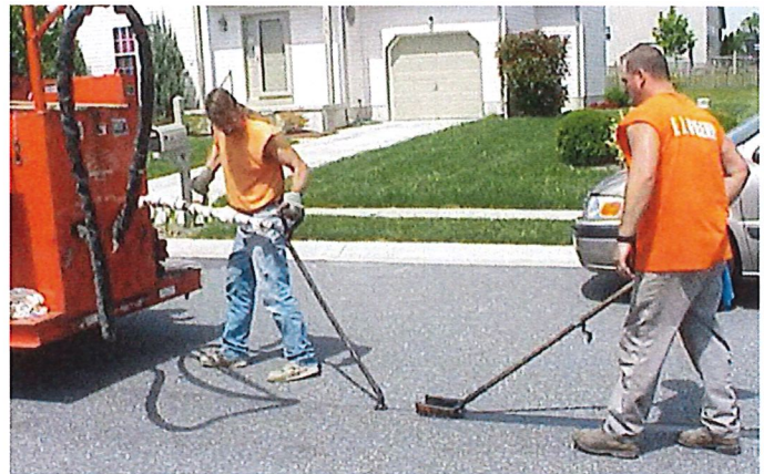
Maintenance: Crack Sealing
