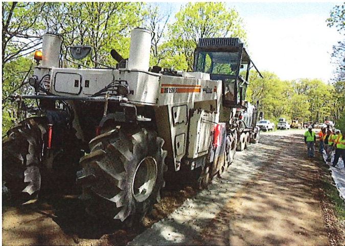
Reconstruction: Full-depth reclamation
